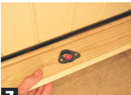
7 Skirting is fitted with Type 1 Fixes, recessed into back. Insert markers and press against panelling
